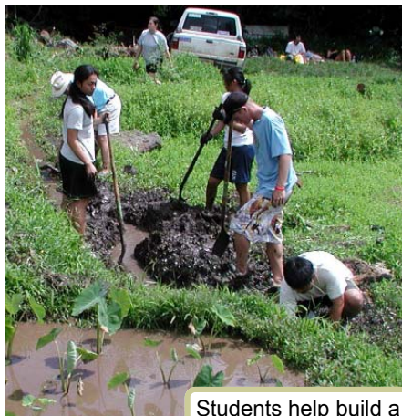
Students help build a new lo'i (Hawaiian taro patch).
